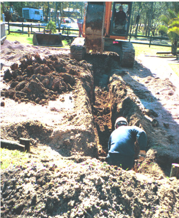
SEWERAGE CONSTRUCTION WORK AT SUTTON PARK ESTATE MEDOWIE continued on page 2
